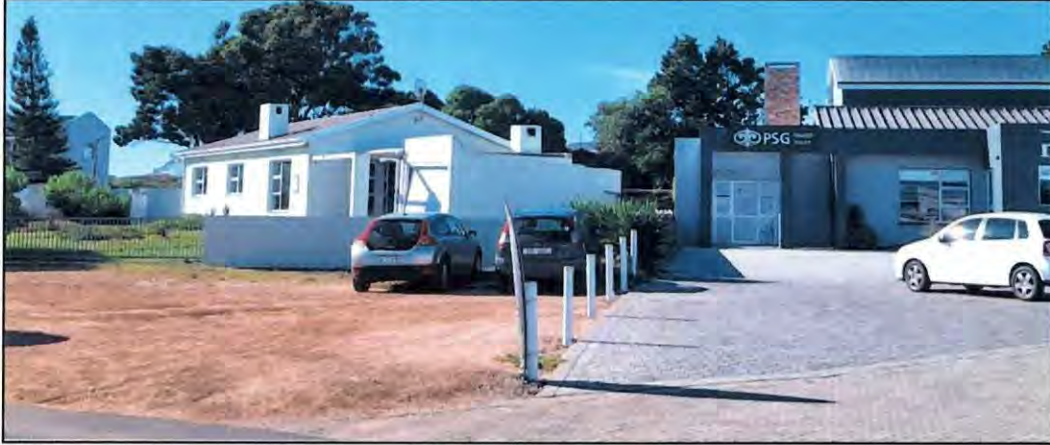
Figure 5: Offices next to Erf 513.
